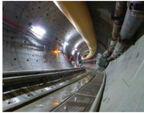
Above: The segmental lining on a finished stretch of the Branch Tunnel
